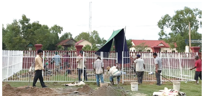
▲ Civil works to construct a foundation, 2020
